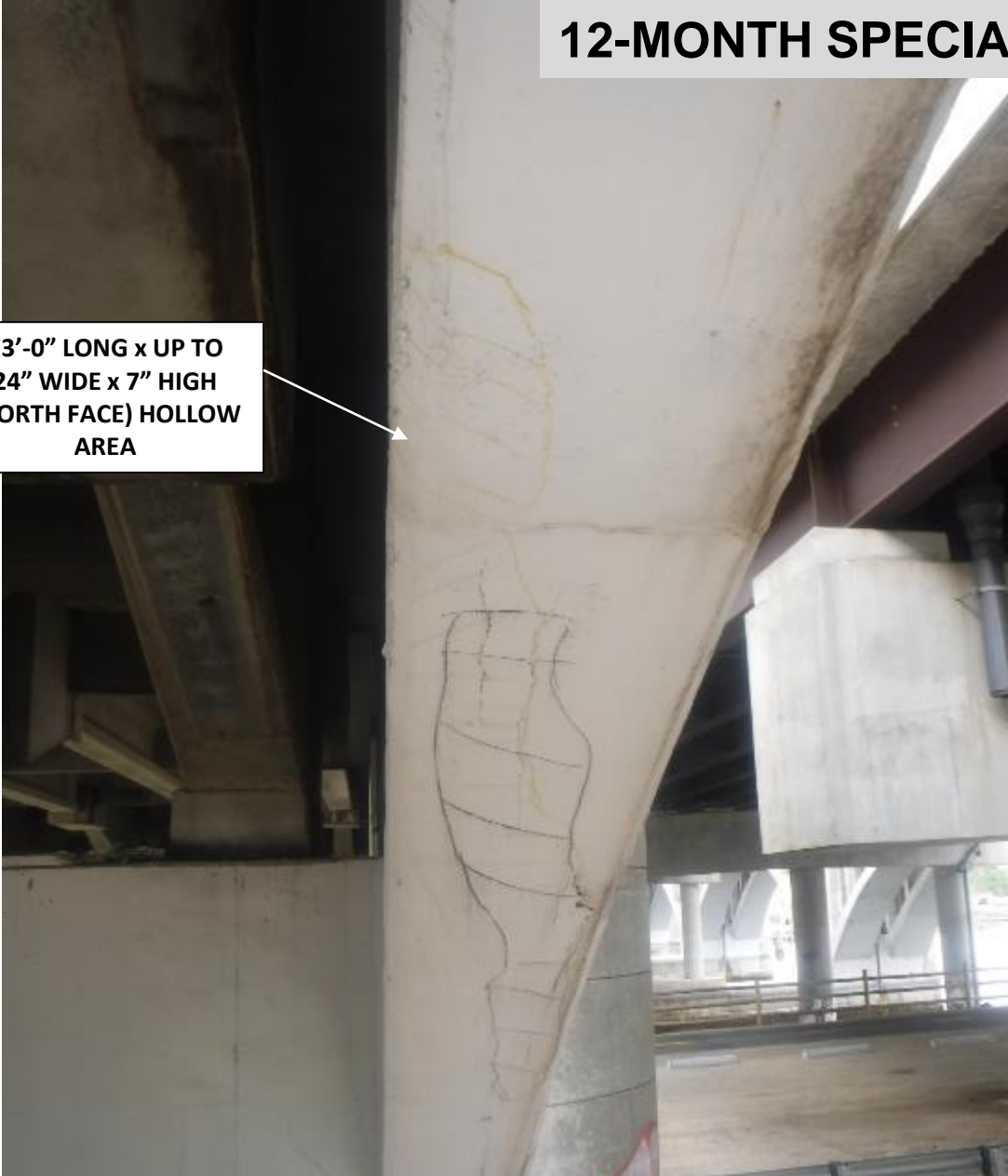
SOUTH ARCH – UNDERSIDE AT EAST JOINT IN SPAN #2
